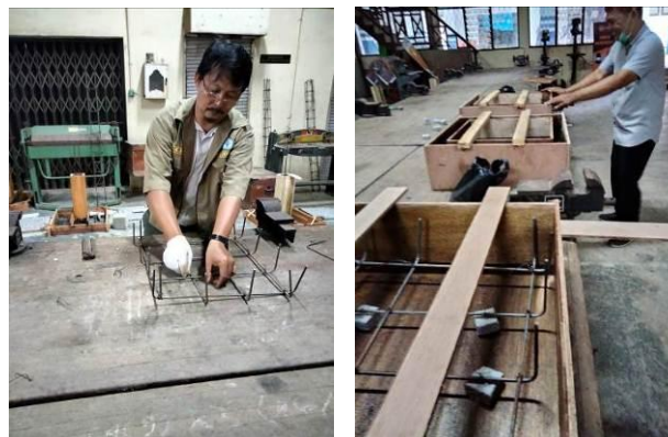
Figure 5: Assembly of reinforcement and formwork
